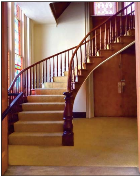
One of the pair of the graceful self-supporting curving stairs in the vestibule of the Presbyterian Church very similar to the ones in the State Capitol.
