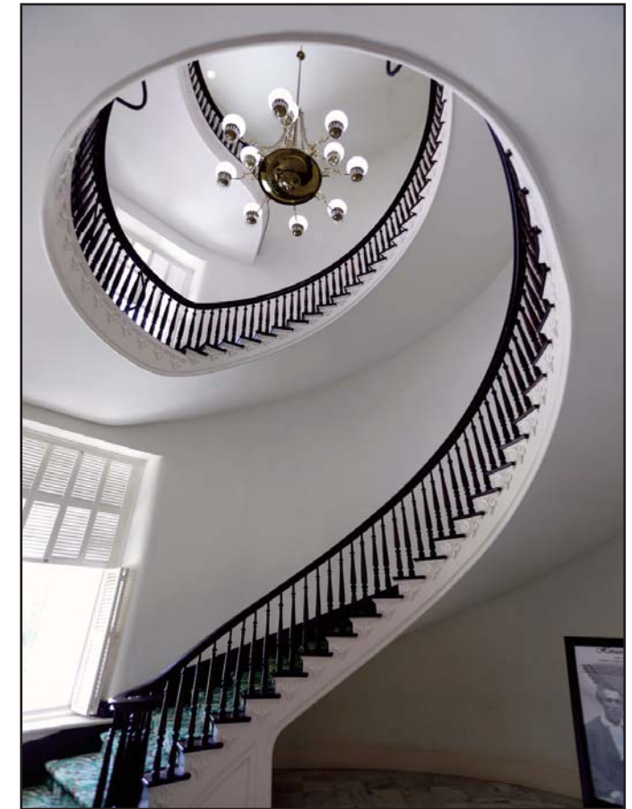
Self-supporting curving stair in Alabama State Capitol - built in 1851 Photo furnished by Tommy Giles
